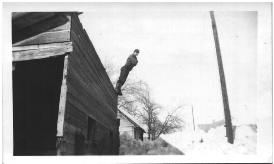
Marvin Tepner getting electrical wire from building to pole on a farm south of town. People were just beginning to get electricity in the country.
